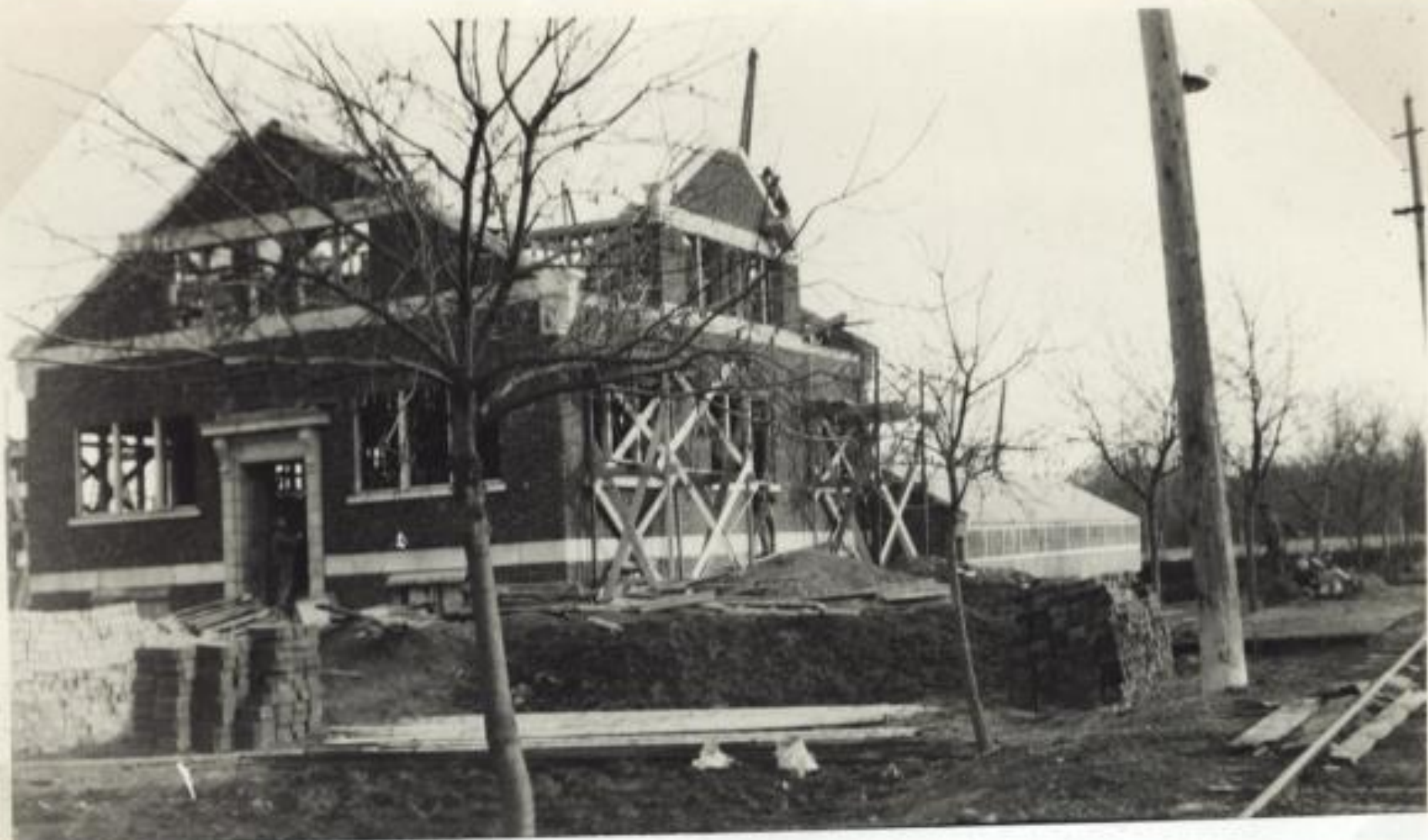
Rust Lab construction
